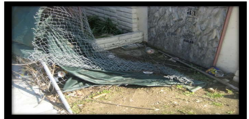
Accessible to unauthorized persons and exhibition of rubbish.
